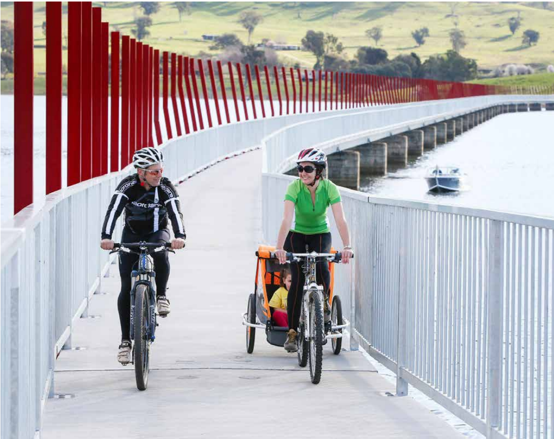
Figure 43. Sandy Creek Bridge, High Country Rail Trail.
