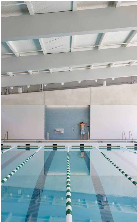
Figure 74. Covered swimming pool, Garfield Centre, San Francisco.
