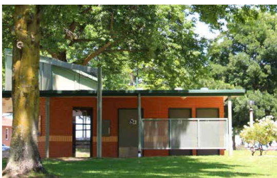
Figure 59. Tallangatta Visitor Information Centre and public toilets.
