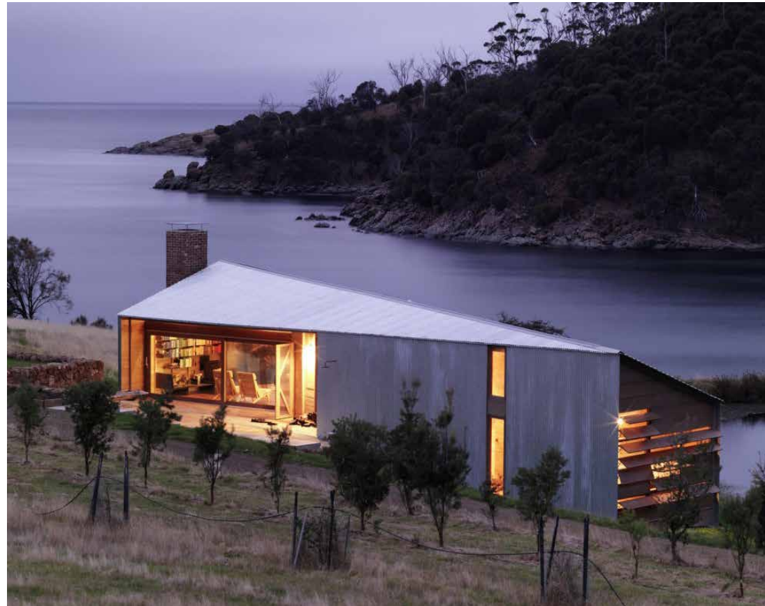
Figure 52. Rural housing, Tasmania.
