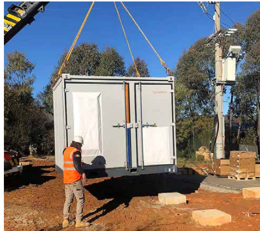
Figure 64. Yackandandah town battery.
