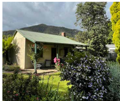
Figure 24. Mitta Mitta residence.
