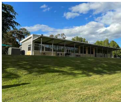
Figure 23. Magorra Park Multi-purpose Centre.
