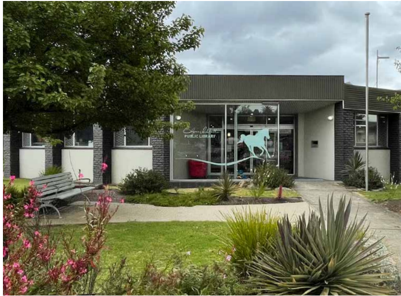
Figure 18. Council offices and library.
