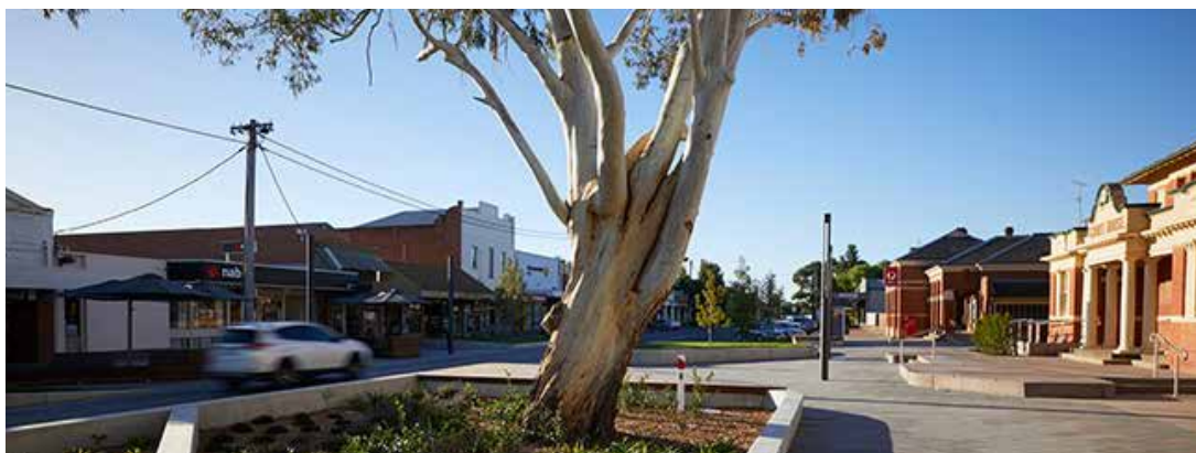
Figure 60. Main street upgrades, Kerang.
