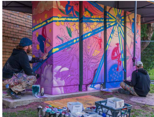
Figure 39. Example of services infrastructure with artwork.
