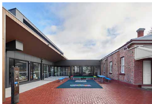
Figure 34. New library at the Former Corryong Junior Campus incorporating heritage buildings.
