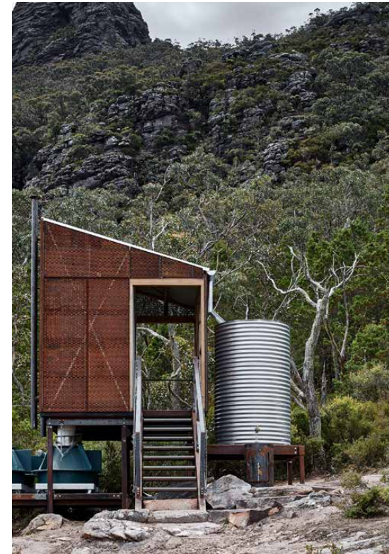
Figure 53. Water collection and septic tanks.
