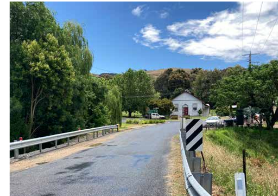
Figure 32. Bridge over Bethanga Creek with Memorial Hall and village centre in the distance.
