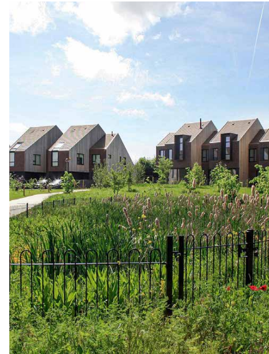
Figure 57. New housing development.
