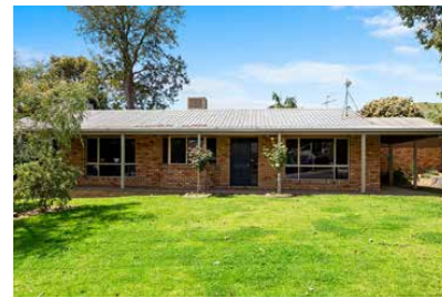
Figure 21. House on Murray Place.
