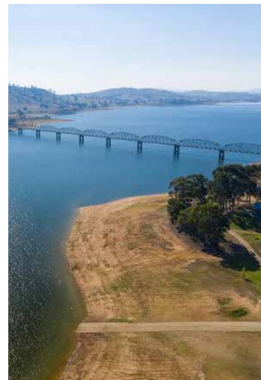
Figure 49. Waterfront restoration to reduce erosion.
